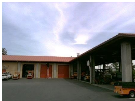
Maintenance Building and Covered Portico
