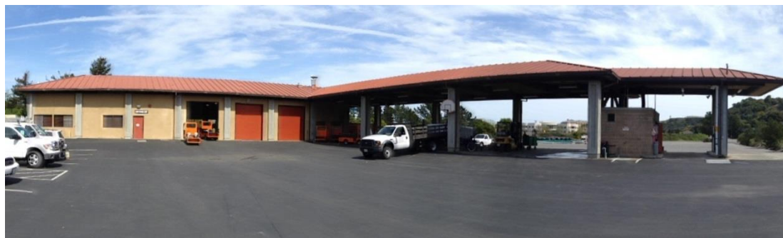
Maintenance Building with standing seam metal roofs.
