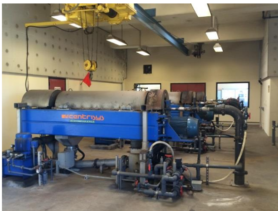
Existing Centrifuges
