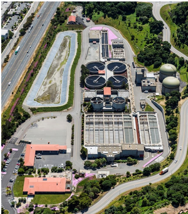
(Clockwise upper left to right): Effluent Storage Pond, Maintenance Annex (red roof behind the pond), Chlorination/Dechlorination Building, Chlorine Contact Tanks, Effluent Pump Station, Secondary Clarifiers, Solids Handling Building, Organic Waste Receiving Facility, Digesters and Digester Building, Aeration Tanks, Biotowers, Primary Clarifiers and Blending Channel, Grit Building, and Headworks. The two orange-roofed buildings in the lower center are the Maintenance Building (top) and the Administration Building (bottom).
